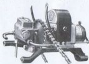
The Duplex Oil Pump, mounted on Magneto Platform, showing one of the two sight-feed regulators.
