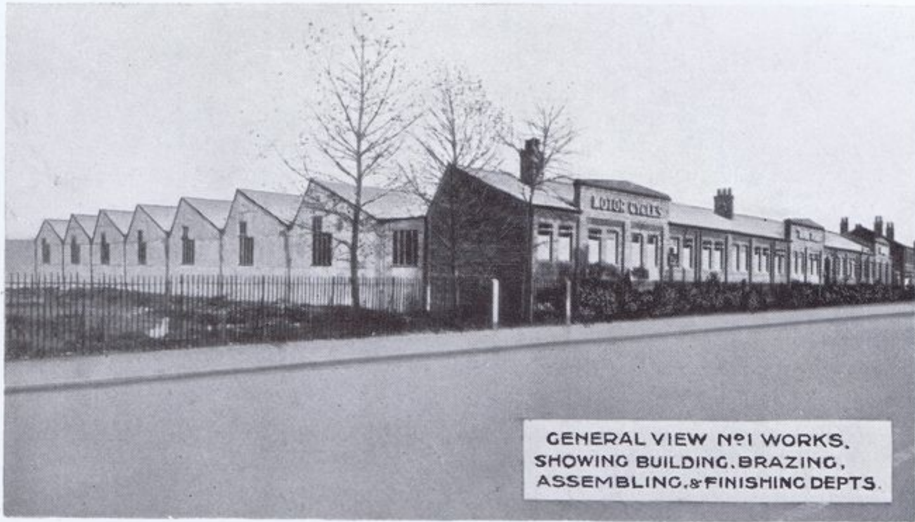
FRONT ELEVATION N° 1 WORKS
