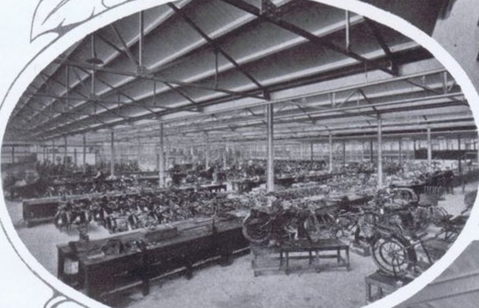
GENERAL VIEW WORKS INTERIOR
